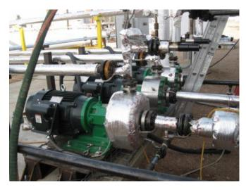
Photo by Magnatex Pumps, Inc. A magnetically driven centrifugal pump used in CL-WGTF.
