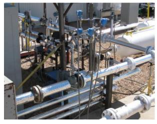
Wet gas meter calibrations are usually done using natural gas, kerosene and water. Increasingly, gas producers are questioning a meter's ability to measure wet gas entrained with the unique liquids found on platforms and wellheads (viscous hydrocarbons, paraffin based/high-wax liquids, sea water, brine solutions, MEG and other custom liquids).
